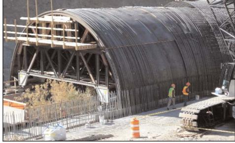
A temporary arch is constructed over Galena Creek, as part of NDOT's I-580 Extension from the Mount Rose Interchange to Bowers Mansion
